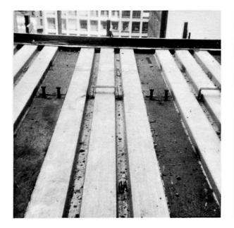
Fig. 11. Category II(b) Form — Special module designed to carry service wiring.
