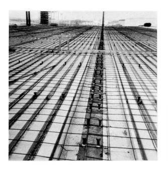
Fig. 13. Category II(b) Form — Overview showing composite beam and girder construction. (Note temperature steel.)
