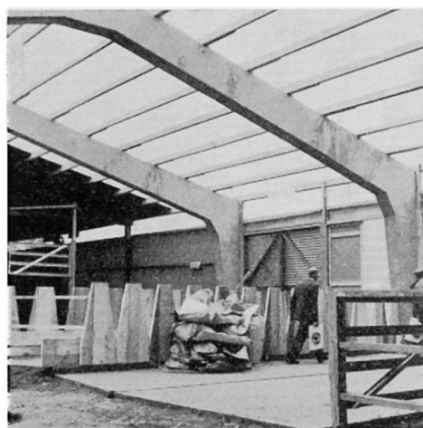
Fig. 13. Two-hinged arches made of three parts. The joints are made as shown in Fig. 5.
