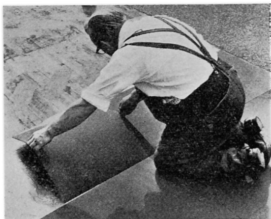
Fig. 5. Laying thin sheeting based on poly-vinyl chloride.
