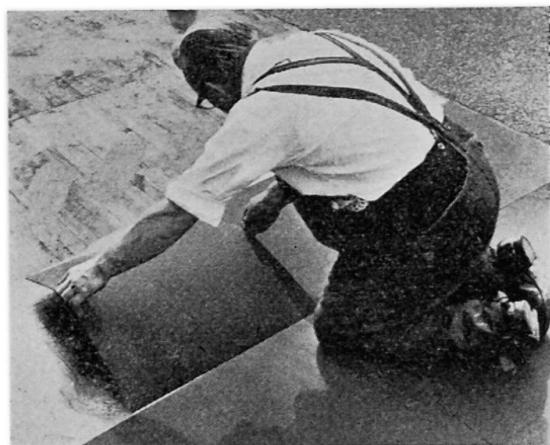
Fig. 5. Laying thin sheeting based on poly-vinyl chloride.
