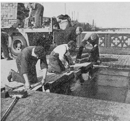
Fig. 4. Laying wood blocks which have been previously coated with an epoxy-resin-based surfacing; Tower Bridge, London, 1962.
