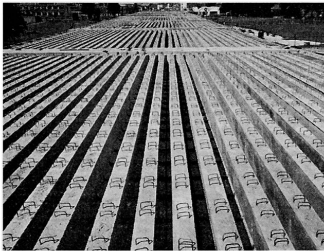
Fig. 7. Prestressed bridge beams in the Chiswick-Langley motorway.
