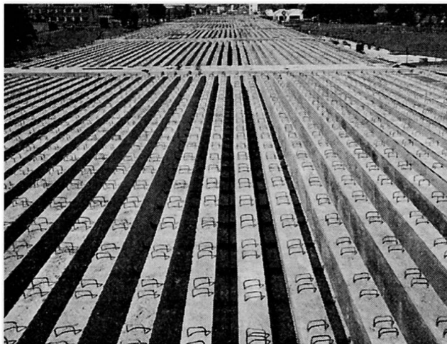
Fig. 7. Prestressed bridge beams in the Chiswick-Langley motorway.
