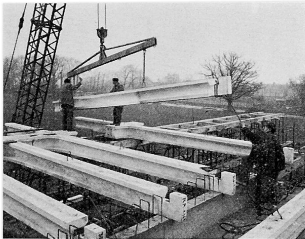
Fig. 5. Cruciform units for a pavilion roof.
