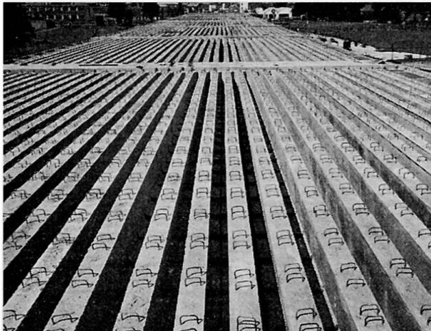
Fig. 7. Prestressed bridge beams in the Chiswick-Langley motorway.
