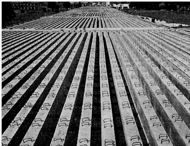
Fig. 7. Prestressed bridge beams in the Chiswick-Langley motorway.
