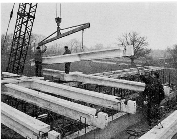
Fig. 5. Cruciform units for a pavilion roof.
