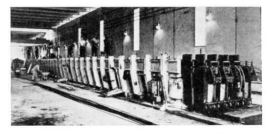
Fig. 4 - Production Machine for Prestressed Cored Slabs.
