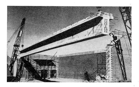
Fig. 3 - Lightweight Aggregate Girder 98 ft. Long.
