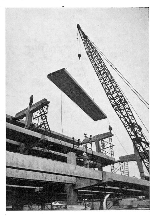
Fig. 5 - Erection of Cored Slabs.
