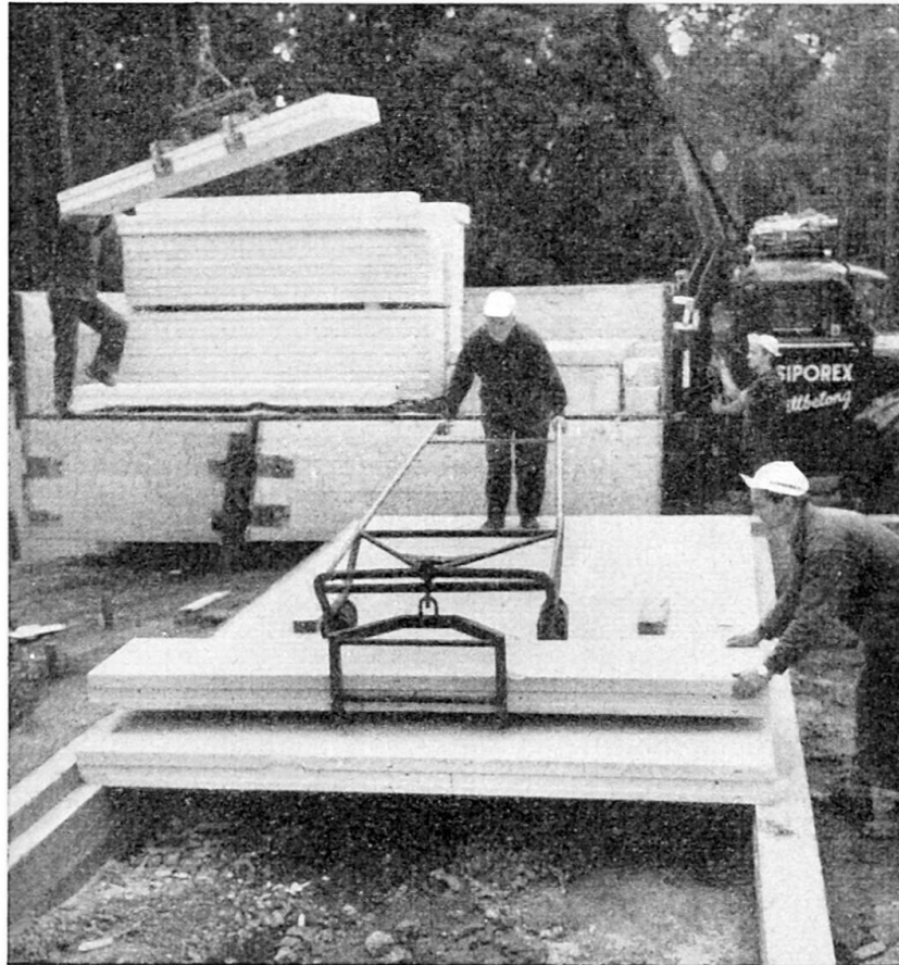
Fig. 11 - Floor panels with groove and tongue.
