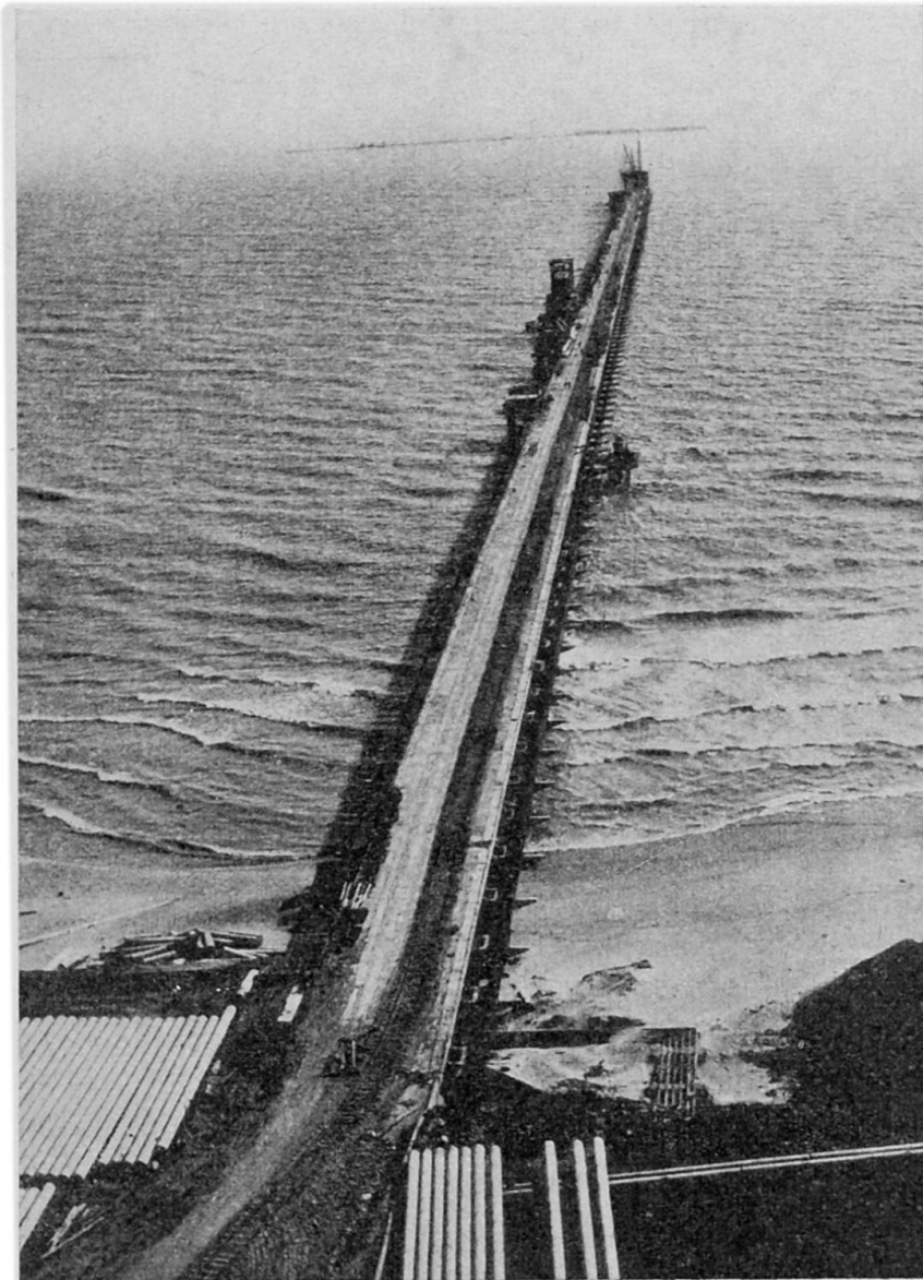
Fig. 17 - ANIC loading dock at Gela, Sicily. Prestressed foundation piles (Impresa Vianini).
