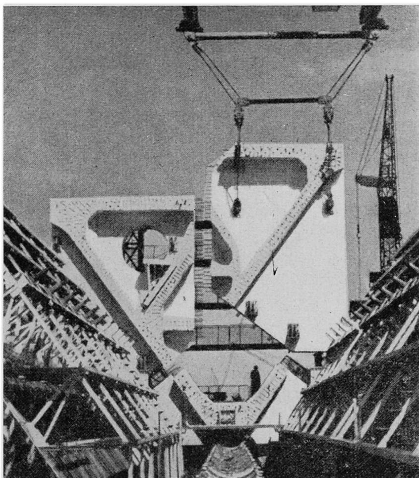
Fig. 9.5 - Placing the three parts of an end-section.
