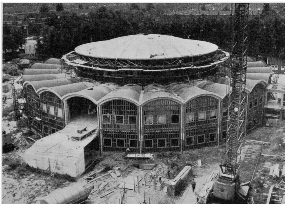
Fig. 7.2 - The rotunda with conical shells and dome.
