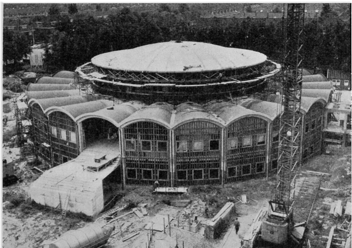
Fig. 7.2 - The rotunda with conical shells and dome.
