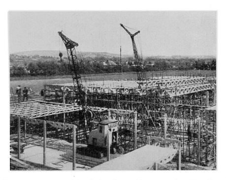
Fig. 8 - Precast concrete units of the Intergrid system for Worthing Secondary Technical School.
