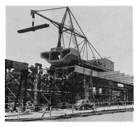
Fig. 11 - Precast concrete units for Hammersmith Flyover.
