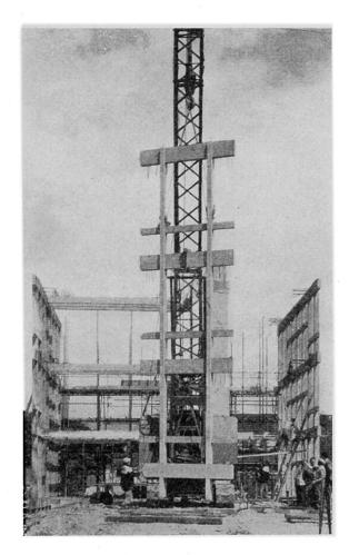
Fig. 6 - H-frame column units being erected for the Marley Tile Co. Ltd.
