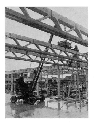
Fig. 7 - Laingspan units being erected for the Alperton School.
