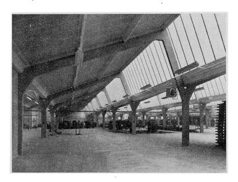
Fig. 5 - Precast northlight framework for factory at Bracknell New Town.
