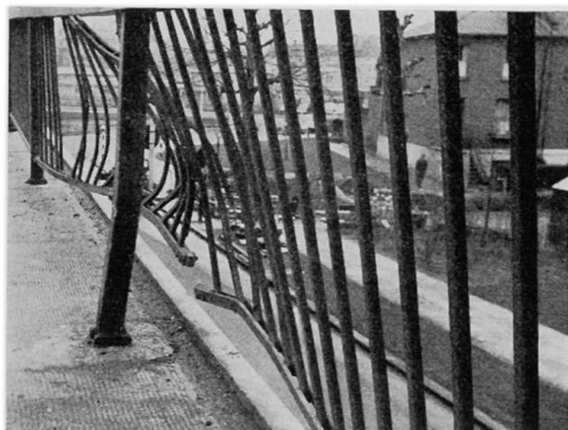
Fig. 10. Damage to bridge parapet railing after impact from sports car.
