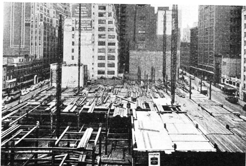
Fig. 13. With several derricks erecting, staggering the time of jumping results in better delivery of steel. Working floors should be completely planked for safety.
