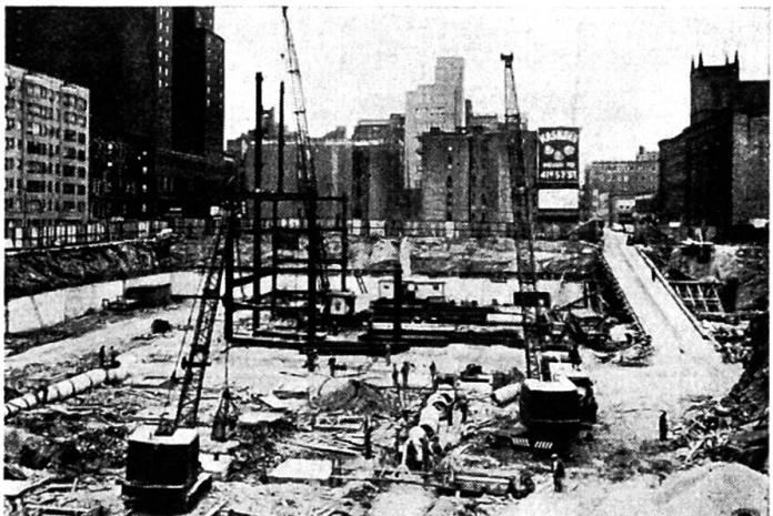
Fig. 3. A ramp is often needed at the site when foundation is considerably below ground level.
