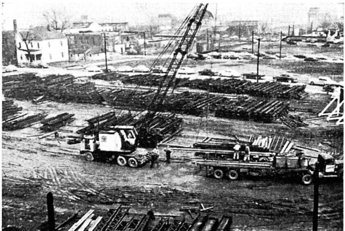
Fig. 2. An unloading or sorting yard is necessary for most efficient tier building erection.
