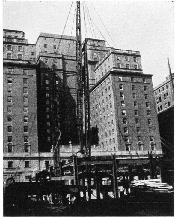
Fig. 7. To jump guy derrick, boom is separated from mast, guyed as a pole to lift mast to upper floor. Mast then picks boom up to itself.
