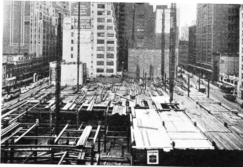
Fig. 13. With several derricks erecting, staggering the time of jumping results in better delivery of steel. Working floors should be completely planked for safety.
