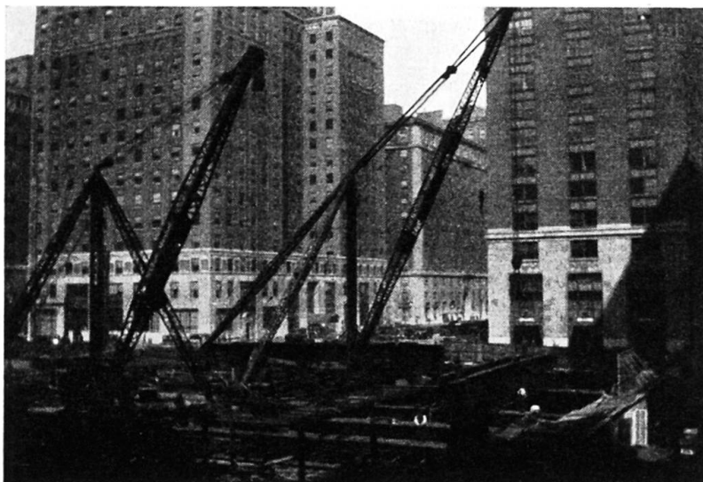
Fig. 14. Stiffleg derricks are sometimes used as travelers to erect heavy steel below street level, then setting up guy derricks for the upper, lighter structure.
