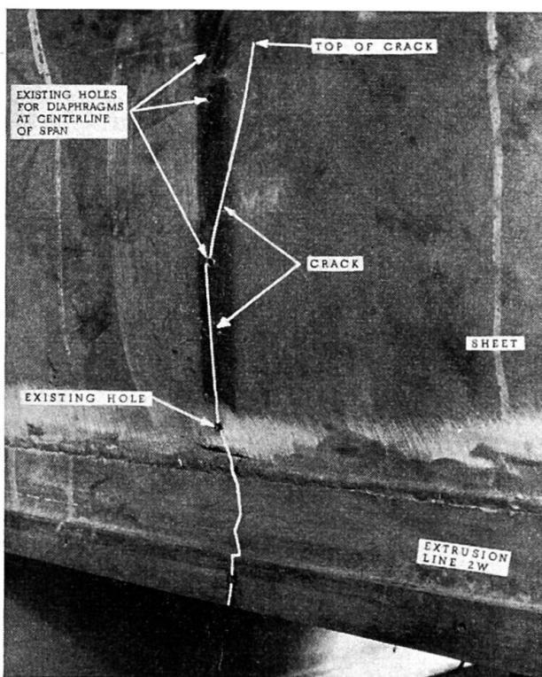
Fig. 6. Crack No. 1.
