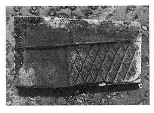
Fig. 3. The Underside of the  $1^{1/2}$ -in. Surfacing Removed From the Junction of the Smooth and Chequered Plate Panels.
