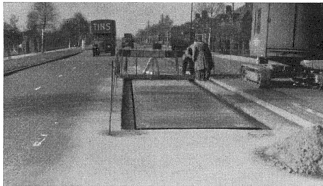
Fig. 2. Panels in Position Prior to Surfacing.
