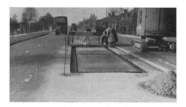
Fig. 2. Panels in Position Prior to Surfacing.
