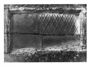
Fig. 4. Deck Plate on the Smooth and Chequered Plate Panels After Removing the 11/2-in. Surfacing. Rusting Can Be Seen Round the Edge of the Plates.
