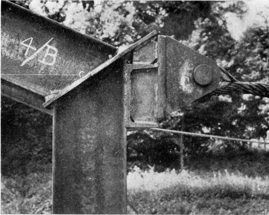
FIG. 3. Joint F, showing side load attachment
