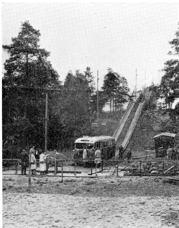
FIG. 5. Slope provided with runway of wood. In the foreground, the parapet fixed in the concrete foundation.
