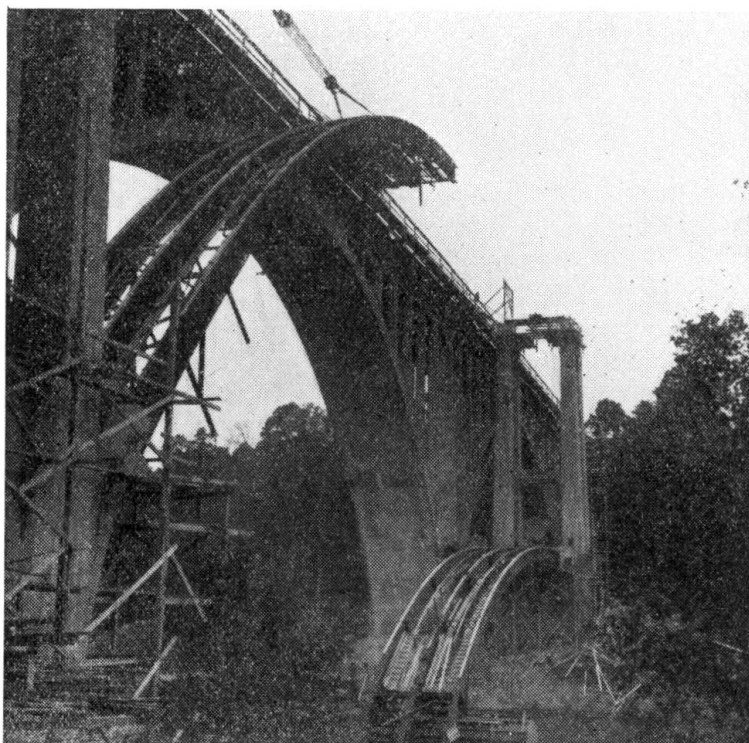
FIG. 6. First part of the arch in its final position, the second being hinged at the abutment
