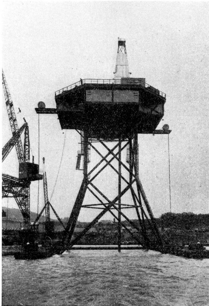
FIG. 8. Tower complete and ready for floating
