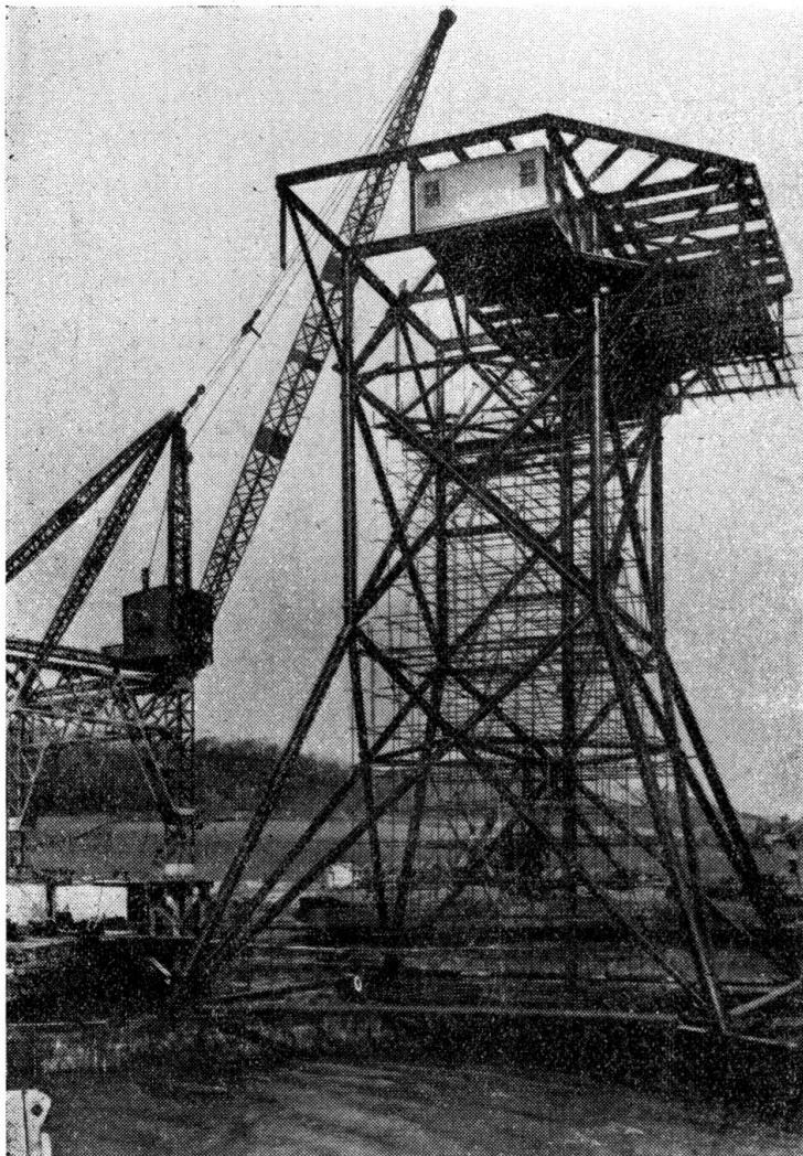
FIG. 6. Assembly of upper decks and accommodation units
