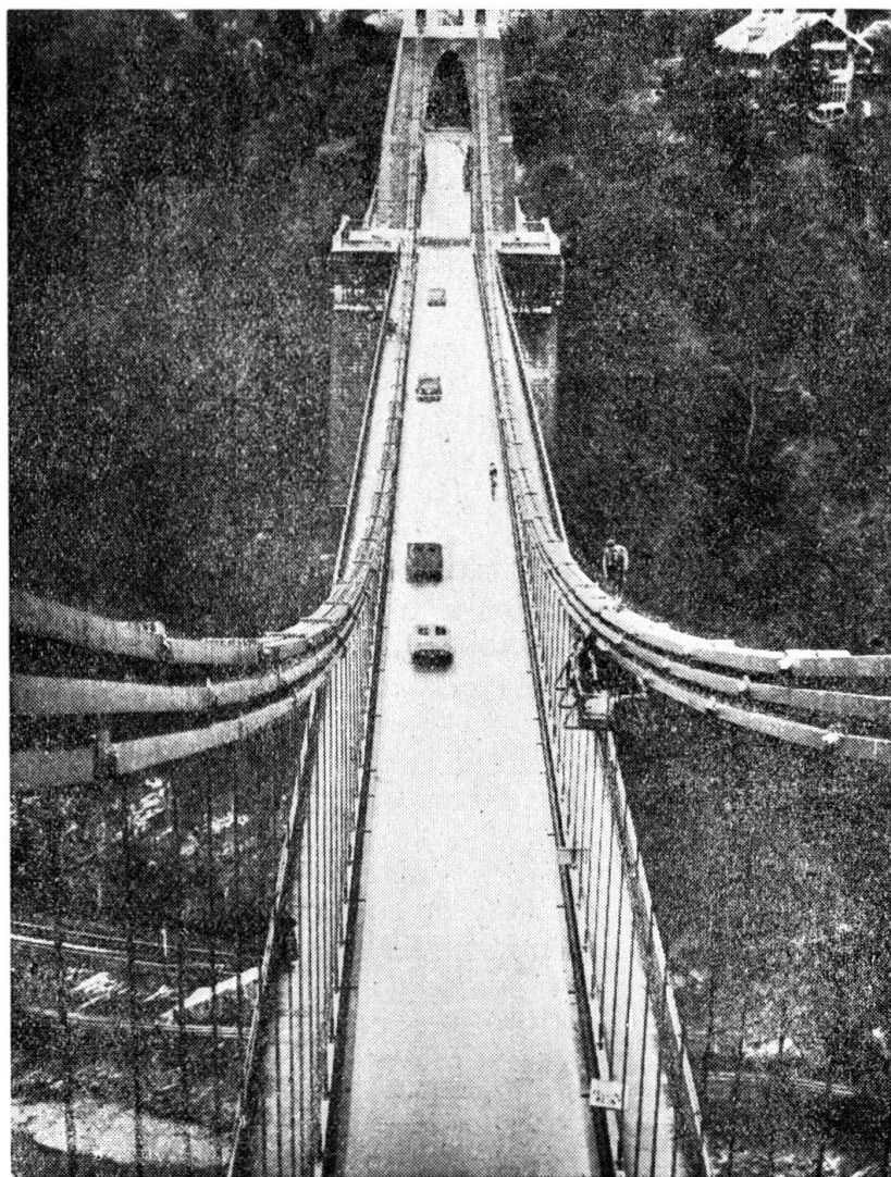
FIG. 1. View of suspension chains «Clifton Bridge». The cradle for metallising is clearly shown. Courtesy of Bristol Metal Spraying & Welding Co. Ltd.
