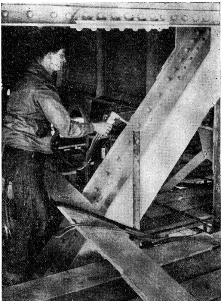
FIG. 5. Zinc spraying the previously sandblasted surface of the Jubilee Bridge, Barrow in Furness
