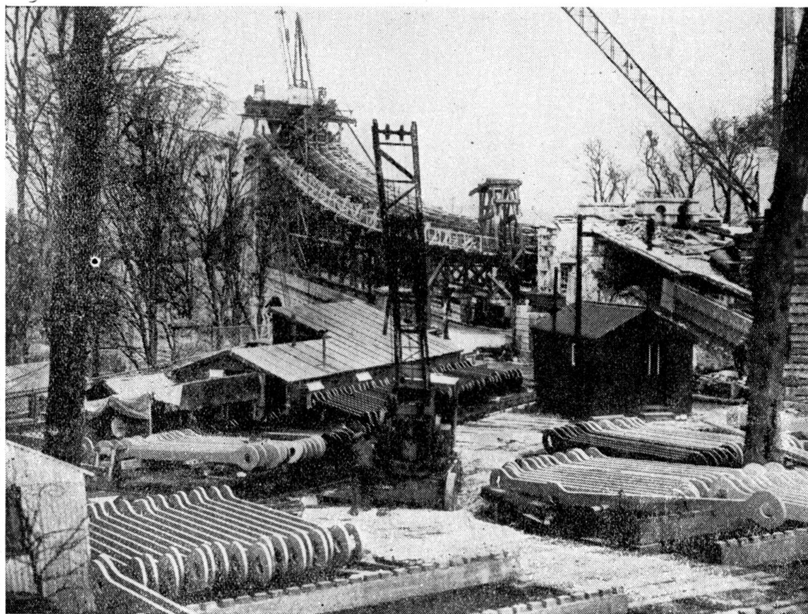
FIG. 6. The sandblasting and zinc spraying of the suspension links of the Menai Straits Bridge in 1939
