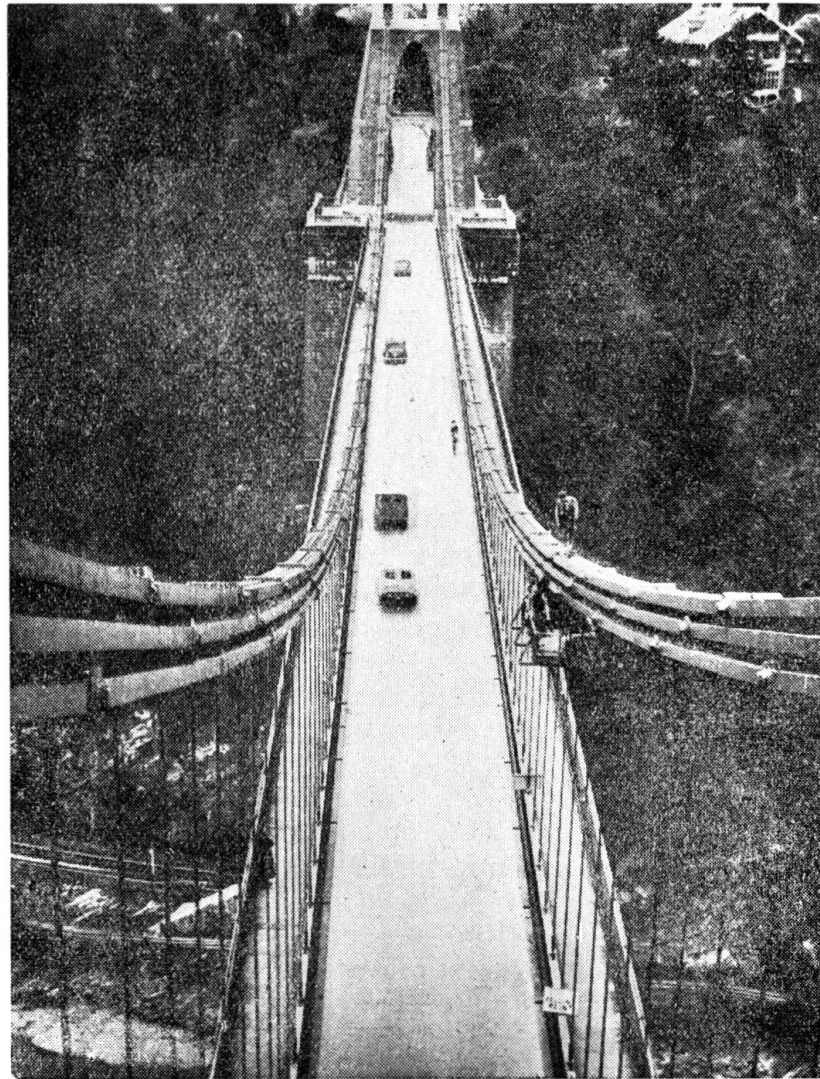
FIG. 1. View of suspension chains «Clifton Bridge». The cradle for metallising is clearly shown. Courtesy of Bristol Metal Spraying & Welding Co. Ltd.
