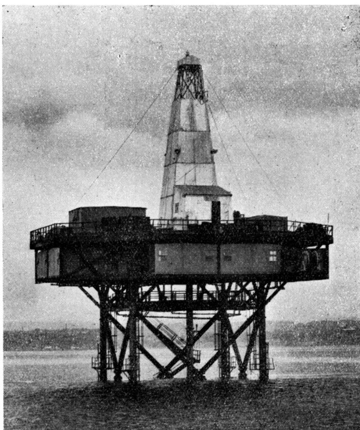
FIG. 10. Tower grounded in its first boring position in the Firth of Forth
