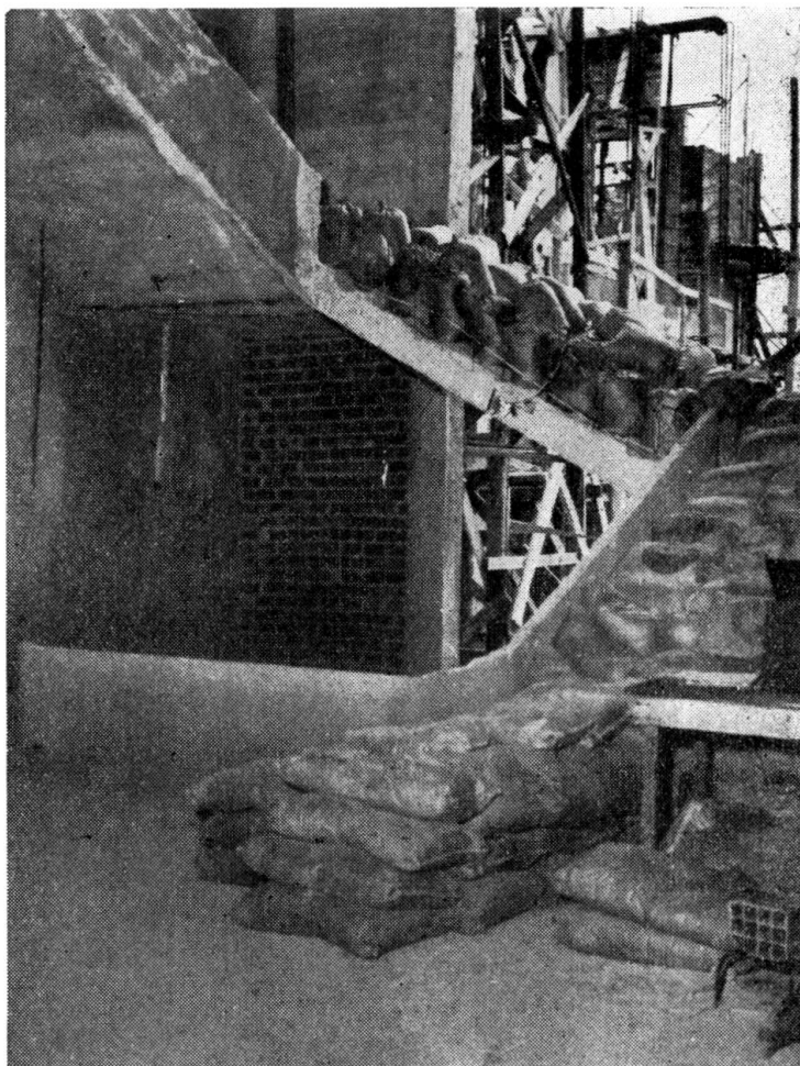
FIG. 8. Application of the uniform load
