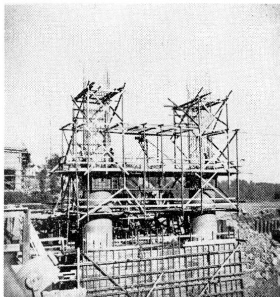
FIG. 11. Columns under construction for a highway bridge across the river Indalsäven at Bergeforsen, Sweden
