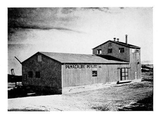
Fig. 9. Utility buildings. Light-gauge steel roofs and walls on structural steel rigid frames. Mass-produced for widths from 16 to 100 ft. (Butler Manuf. Co.)
