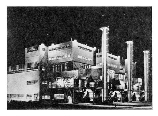
Fig. 14. Electric power plant. Light-gauge steel wall, floor, and roof panels on heavy steel frame (Detroit Steel Products Co.)
