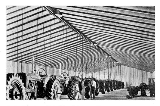
Fig. 10. Frameless utility building, 50 ft. span, with tractors suspended from ridge member (average ridge load 320 lb./ft.) (Behlen Manuf. Co.)
