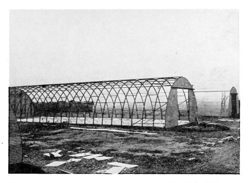
Fig. 8. Quonset Huts, mass-produced for spans from 20 to 40 ft. Light-gauge steel arches, corrugated sheet (Stran Steel Division, Great Lakes Steel Corp.)
