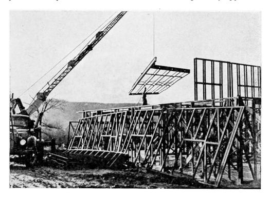
Fig. 12. Erection of prefabricated wall and floor panels for two-storey apartment houses (Stran Steel Division, Great Lakes Steel Corp.)
