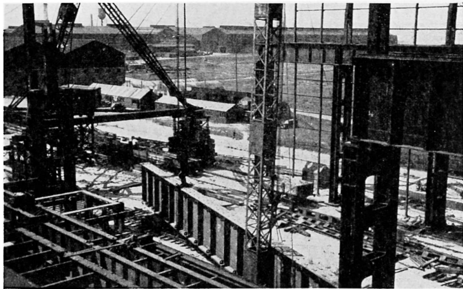
Fig. 10. 100-ton welded girder being lifted by a derrick crane and a derrick mast
