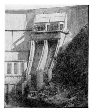
Fig. 13. Spillway of Castelo do Bode Dam
