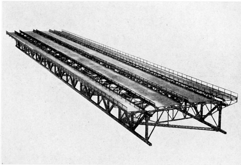
Fig. 5. Sectional model of design proposed for the Severn Bridge (1/32-scale)
