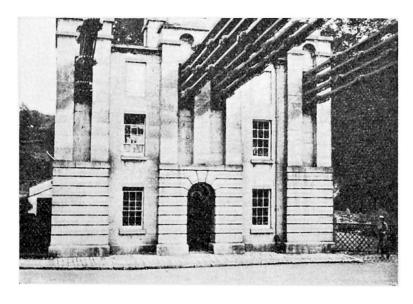
**Fig. 4.** Old chains entering the anchorage on the Welsh side.
