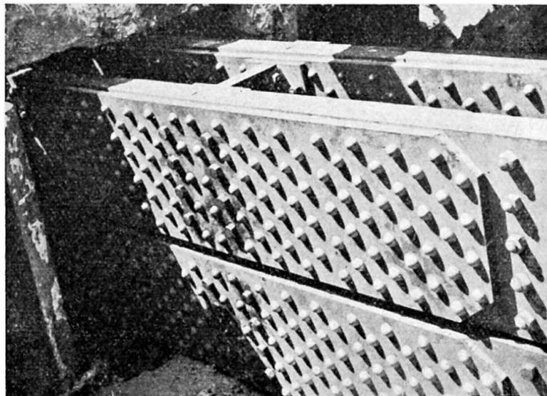
**Fig. 7.** Steel plate extension of the new eyebar chains which were designed to slide down the anchorage tunnels and to be concreted in solid instead of painted and left exposed as were the underground eyebar extensions in the old structure.
