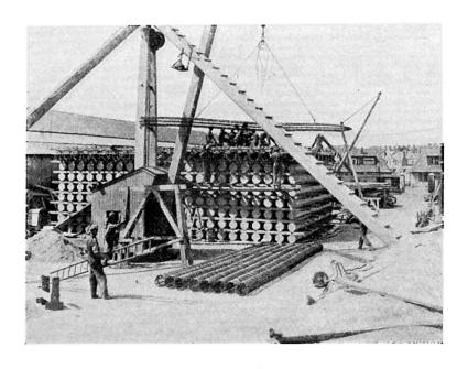
Fig. 7. Fixing reinforcement for piles in casting yard showing stacking of piles.
