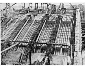
Fig. 13. Centre span reinforcement prior to concreting.
