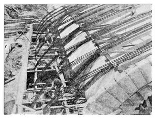
Fig. 12. Reinforcement in arch ribs.
