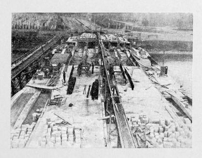
Fig. 15. General view with roadway deck in progress.
