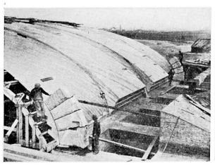
Fig. 10. South Abutment showing first four voussoirs in position.
