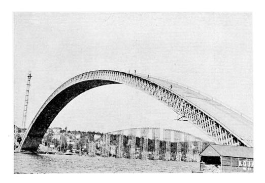
Fig. 6. Freely suspended timber centering.
