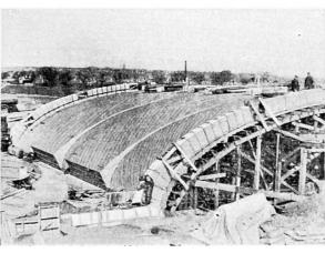
Fig. 11. South Arch span with voussoirs in position and temporary gaps formed.
