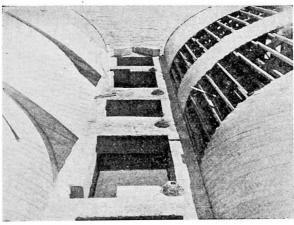
Fig. 9. South Pier. Arch shuttering in progress.
