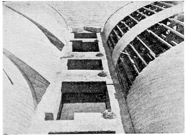
**Fig. 9.** South Pier. Arch shuttering in progress.
