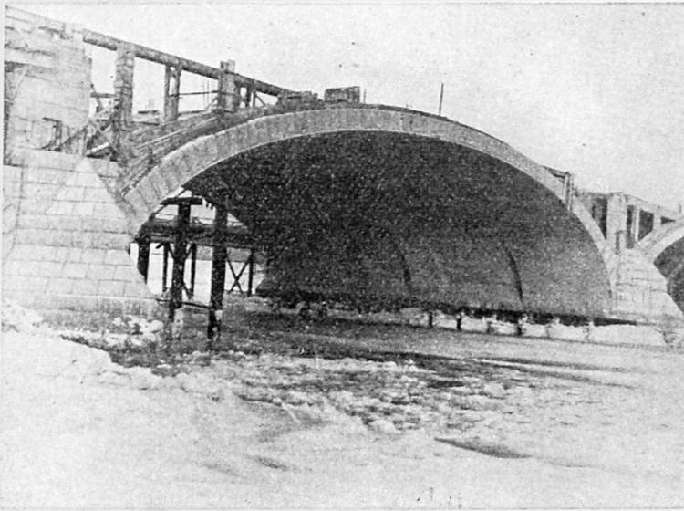
**Fig. 14.** Centre span arch with centering removed.
