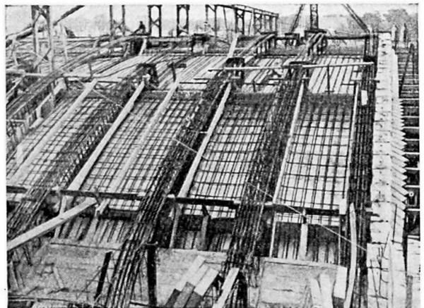
**Fig. 13.** Centre span reinforcement prior to concreting.
