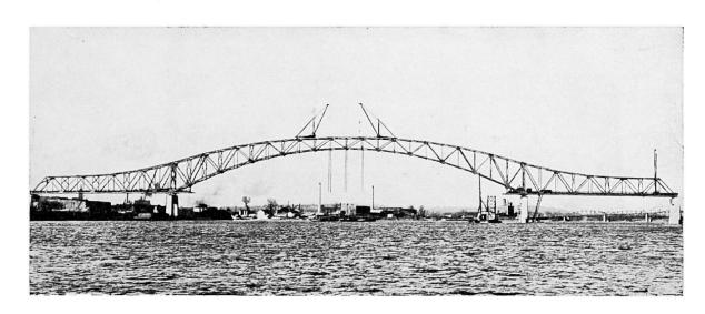
Fig. 7. Arch span fully connected.
