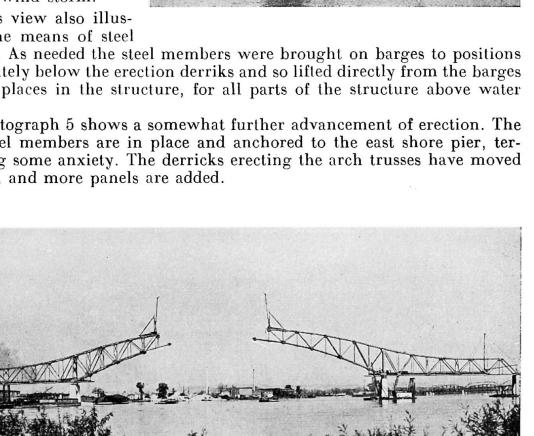
Fig. 5. Further advanced cantilever erection.
