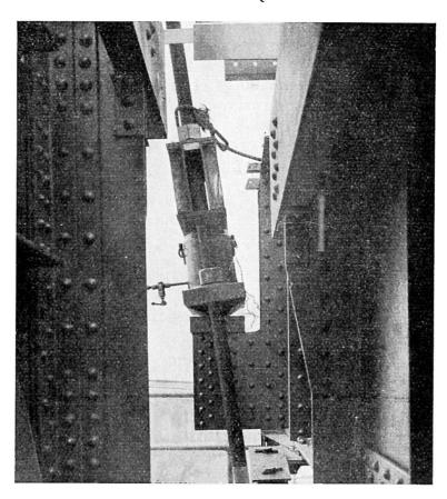
**Fig. 8.** Details provided for lowering and raising the ends of the spans (jack and tic-down bolts).
