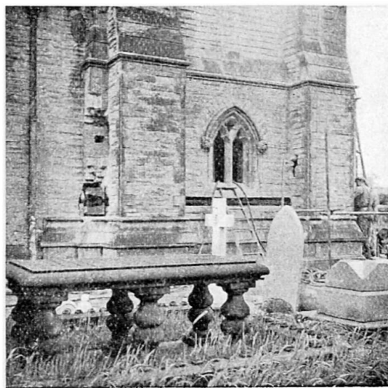
Fig. 4. Chase in the outer wall, with wires before tensioning.
