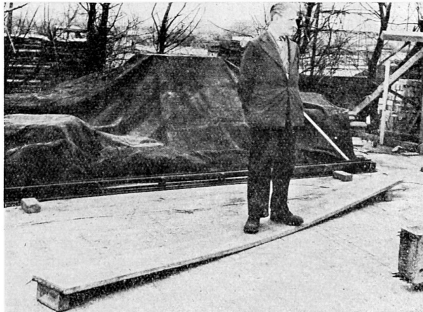
Fig. 3. Prestressed concrete plank 1\frac{1}{4}'' thick, 12 ft span.
