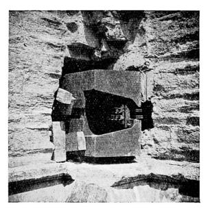
Fig. 7. Strongback with anchorages at one end of the chase (see fig. 4).
