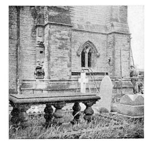
Fig. 3. Chase in the inner wall, where the opening had been bricked up.
