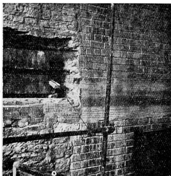
**Fig. 9.** Chase in inner wall (see fig. 3) filled with cement mortar after tensioning.
