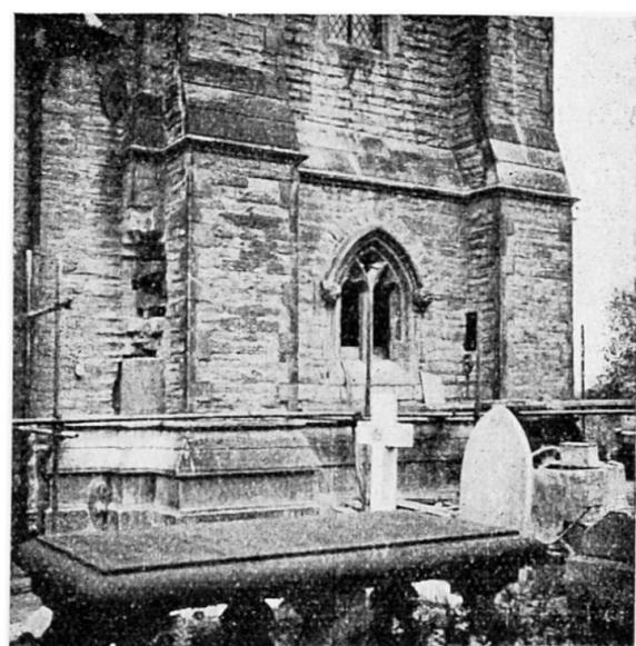
**Fig. 10.** The South side (see fig. 4) after replacing the stone covering, but before tensioning the wires in the Eastern and Western walls respectively.
