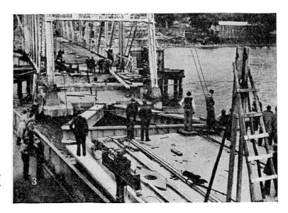
**Fig. 2.** View of the three-leg link of welded plate girder design.
