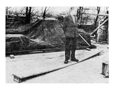
Fig. 3. Prestressed concrete plank 1 1/4" thick, 12 ft span.
