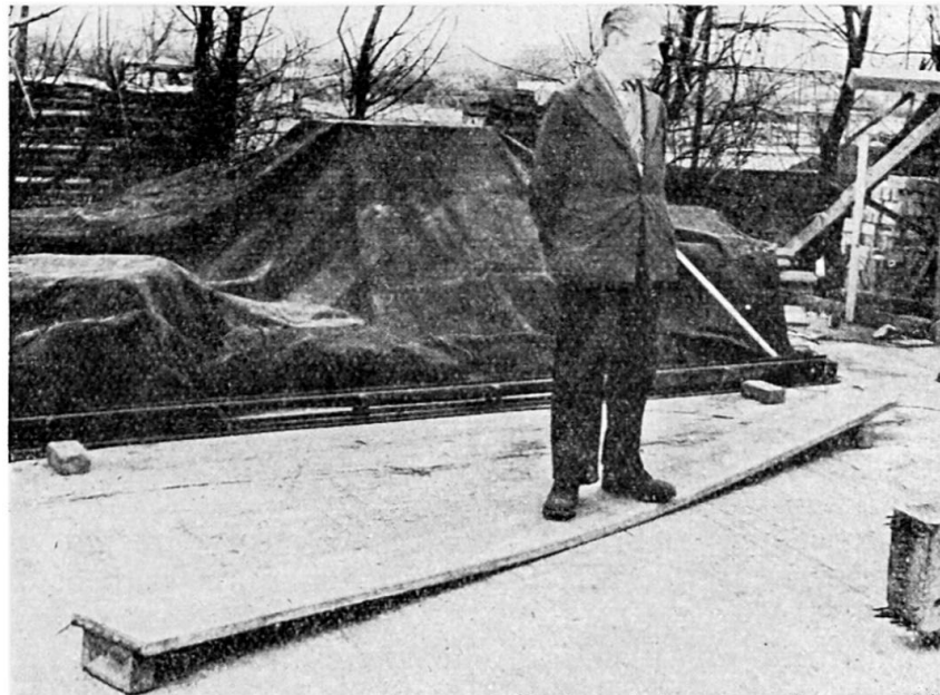
Fig. 3. Prestressed concrete plank 1\frac{1}{4}'' thick, 12 ft span.
