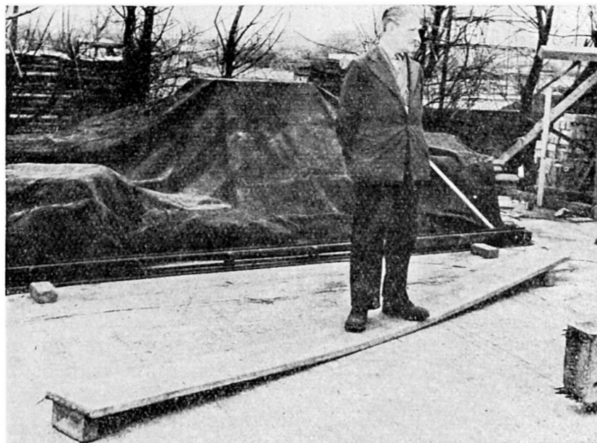
Fig. 3. Prestressed concrete plank 1\frac{1}{4}" thick, 12 ft span.
