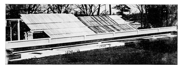
Fig. 1. Prestressed concrete joist. Depth-span ratio 1:45.
