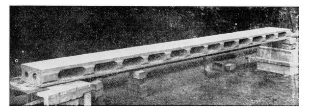
Fig. 2. Prestressed concrete hollow floor unit.
