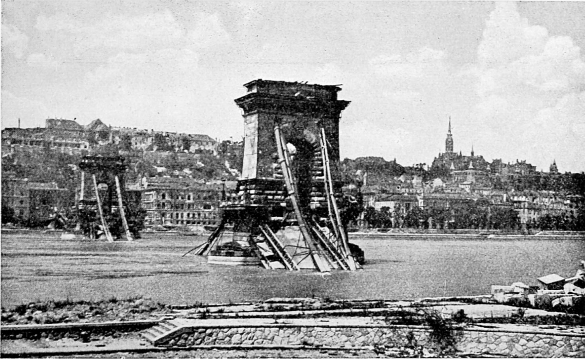
Fig. 4. View of the blown up « Chain-bridge » Budapest.
