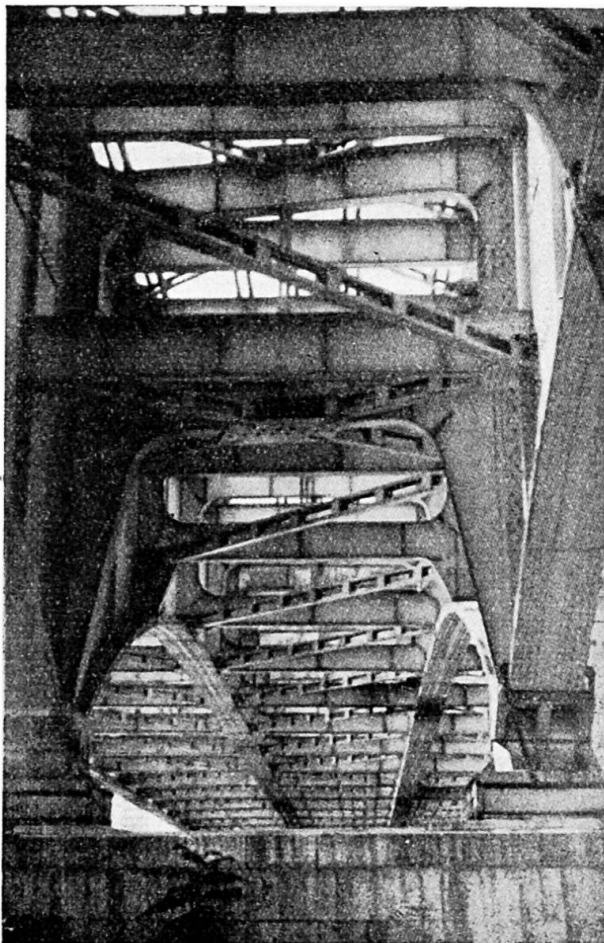
Fig. 2. View of the steel construction of the Arpád-bridge showing welded elements from underneath.
