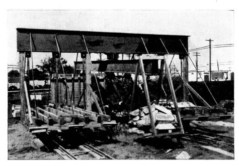
Fig. 1. 60-ton soil testing apparatus.
