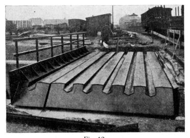
Fig. 12. Schröder-type floor.
