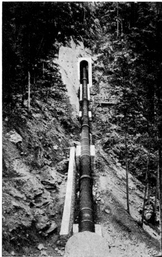
Fig. 4. Armoured portion of entering inclined gallery at level 1220.
