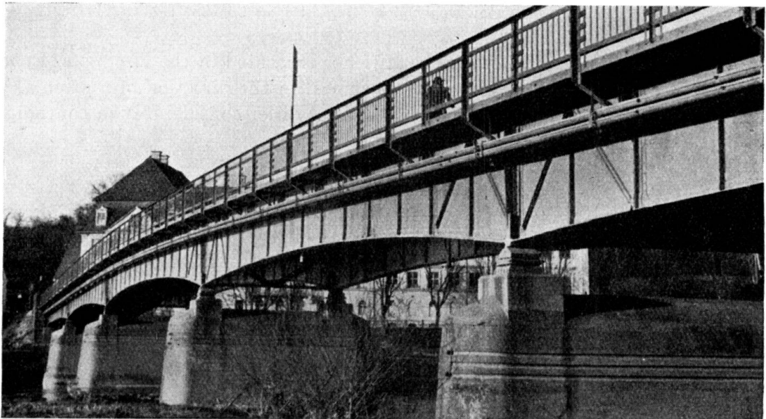
Fig. 6. Road Bridge over the Danube near Donauwörth (largest span 32 m, 1876).
