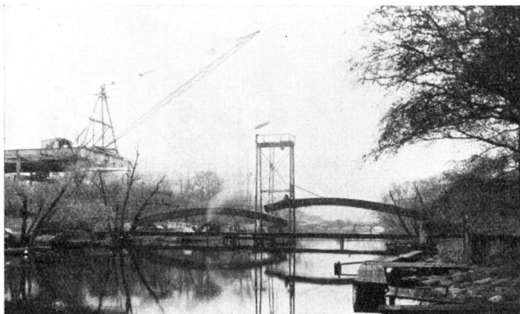
Fig. 14. Pålssund Bridge. Erecting the arches.
