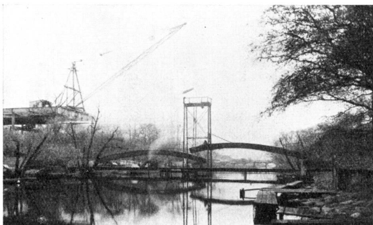
Fig. 14. Pålssund Bridge. Erecting the arches.
