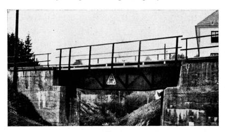
$\label{eq:Fig. 1.} {\rm Fig.~1.}$  Electrically welded railway bridge at Weiz.
