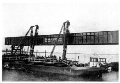
$$\operatorname{Fig.}\ 1.$$  Transporting welded plate girders of 54 m length.
